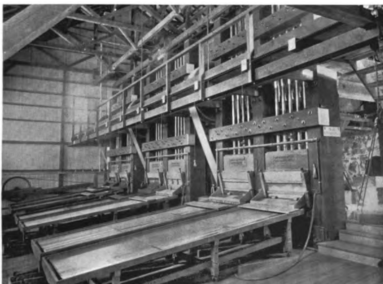
BATTERY ROOM, YELLOW ASTER MILL, RANDBURG.
