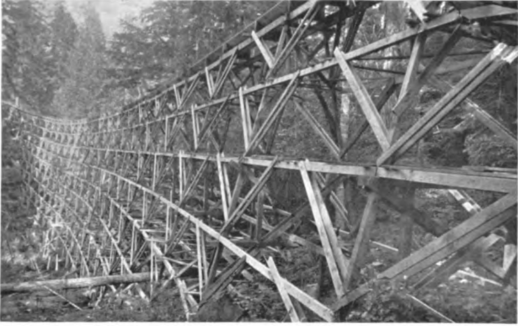
HIGH TRESTLE ON FLUME OF THE BOOTH-KELLY LUMBER CO., SAGINAW, OREGON.
