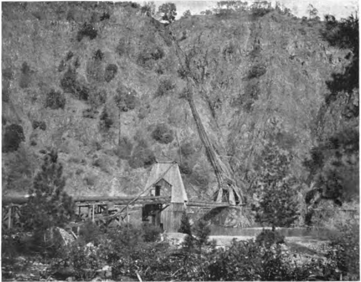
SUSPENSION BRIDGE ACROSS TRINITY RIVER, AT JUNCTION CITY. Carries a Pipe-Line for 3,000 inches of Water under 500 feet Head. Bridge is 350 feet Span. Cables are 620 feet long, 5 inches in diameter, and weigh 11 tons each.
