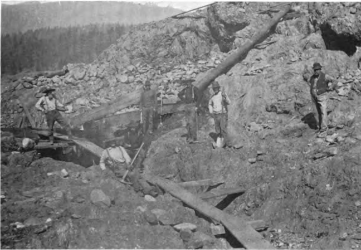
CLEANING BEDROCK AT THE SPANISH RANCH HYDRAULIC MINE, PLUMAS COUNTY.
