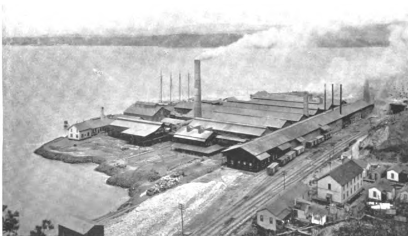
Selby Smelting and Lead Company's Works at Vallejo Junction.
