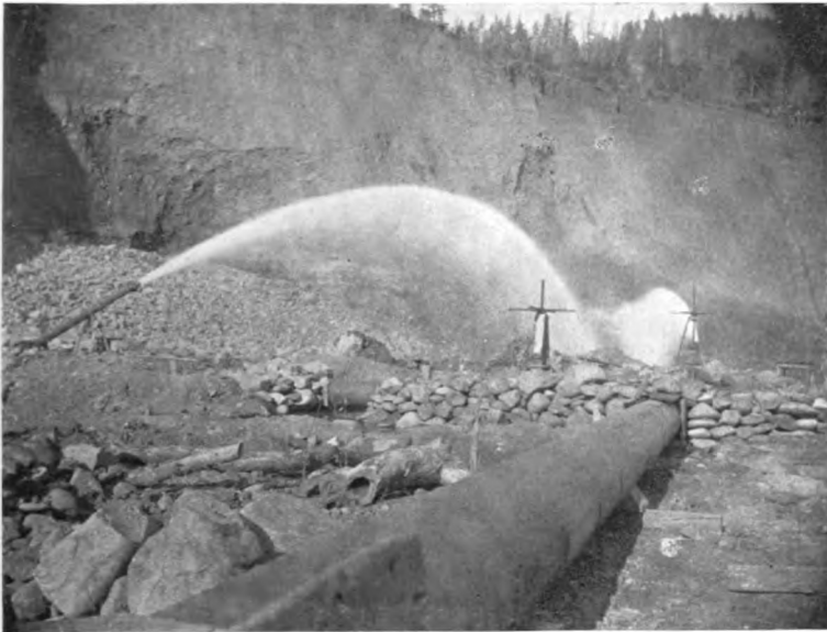
HYDRAULICKING ON THE TRINITY RIVER, NEAR JUNCTION CITY.
