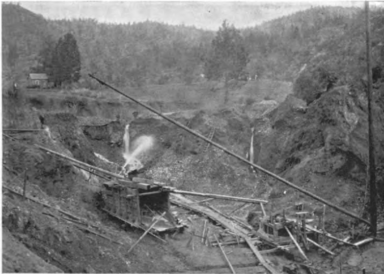
HYDRAULIC MINING IN TUOLUMNE COUNTY.
