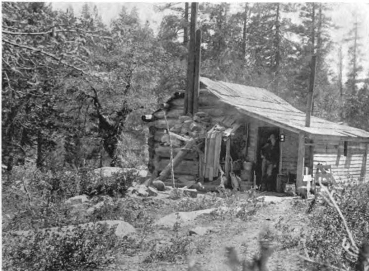
TYPICAL MINER'S CABIN IN REMOTE MINING REGION, PLACER COUNTY.
