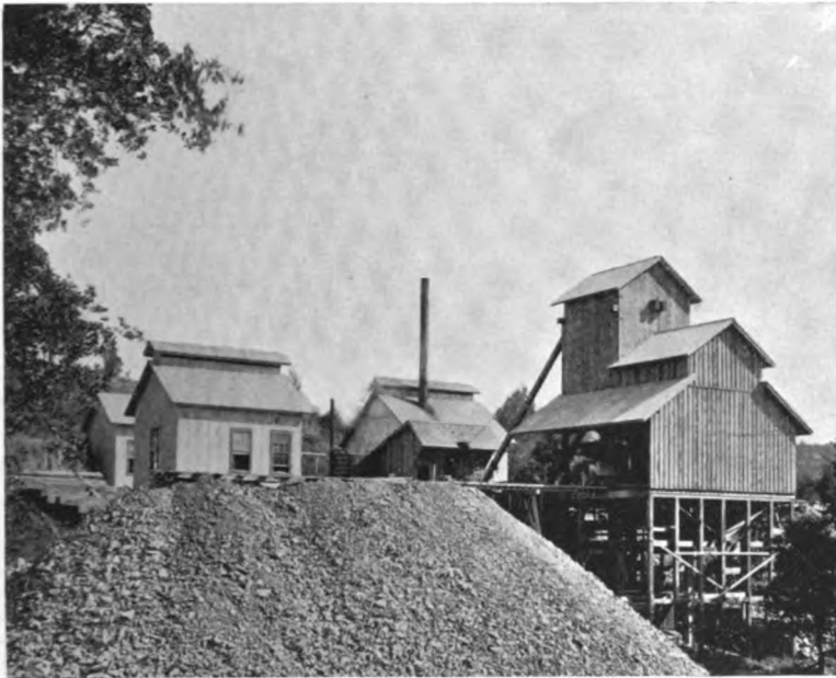
THE SURFACE PLANT AT THE EAST OR NEW SHAFT, KENNEDY MINE.
