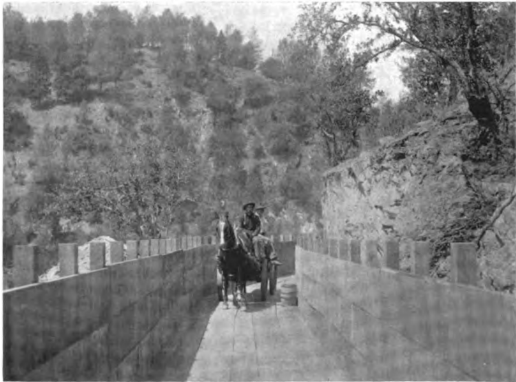
FLUME TO CARRY 600 MINER'S INCHES OF WATER FROM THE STANISLAUS RIVER TO THE 120-STAMP MILL AT THE MELONES MINE.
