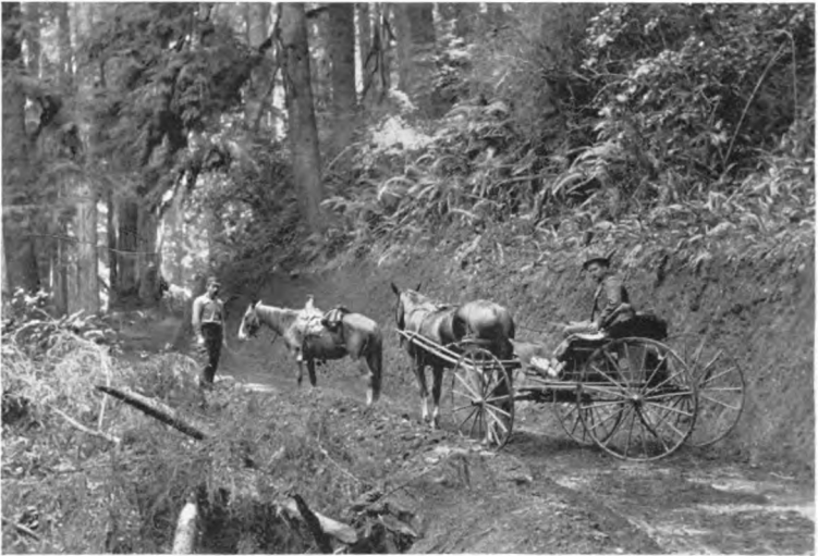
EN ROUTE TO THE BEACH MINES, HUMBOLDT COUNTY.
