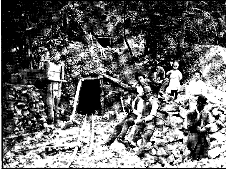
TUNNEL ENTRANCES—STERLING QUARTZ MINE
