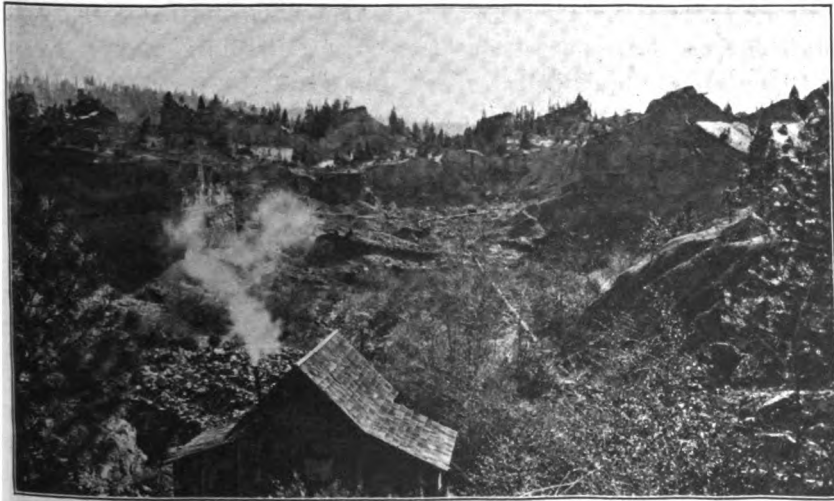
Photo No. 20. Stewart Gravel Mine, near Gold Run. The tailings pile, from the drift workings, may be seen just back of the superintendent's house.
