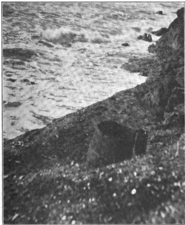
Well drilled in bituminous shales at Carpinteria. Filled with liquid asphalt.
