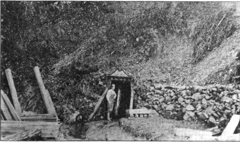
Photo No. 9.—Tunnel entrance to Lucky John drift mine near Paradise.
