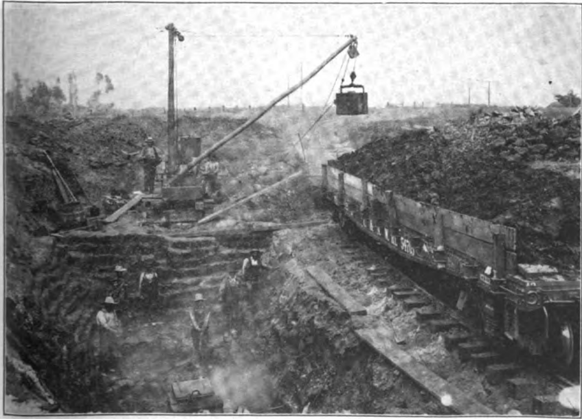
Mining bituminous sands at Higgins Mine for paving Goleta Road. Photo by A. Sattler.
