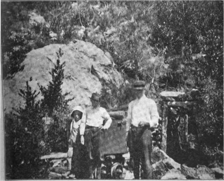
Outcrop and tunnel, Doty Mine, San Luis Obispo County. Photo by E. W. Carson.
