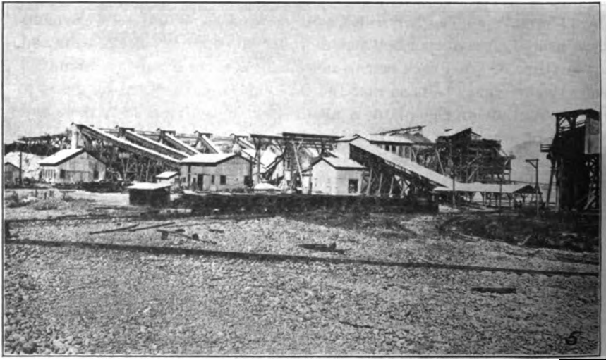
Photo No. 46. Natoma Rock Crushing Plant near Fair Oaks.
