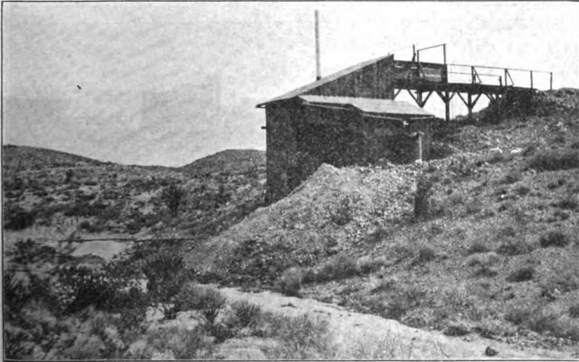
Photo No. 32. Dry concentration mill of Lombard and Main, Signal District, 8 miles north of Goffs.
