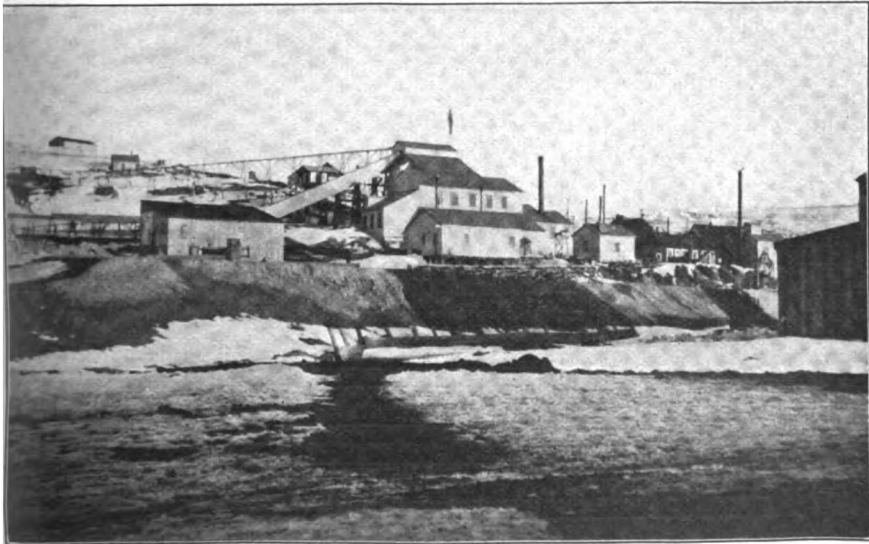
Mill of Standard Consolidated Mine at Bodie. Incline at left is for ore cars. High-line flume conveys tailings to cyanide plant. Photo by Walter W. Bradley.
