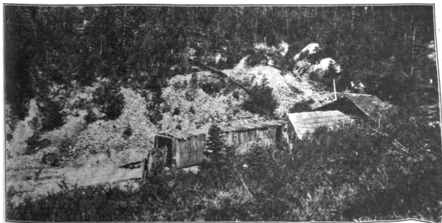
Photo 14. Tunnel entrance to Monumental Mine, Canada Hill District, Placer County.
