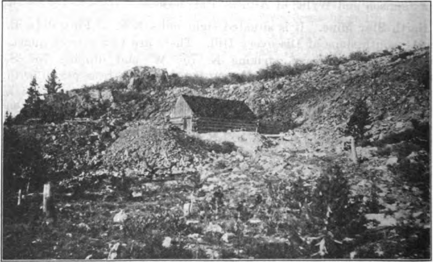
Sunshine tunnel, High Grade mining district, showing typical "rock piles" of High Grade Hill.
