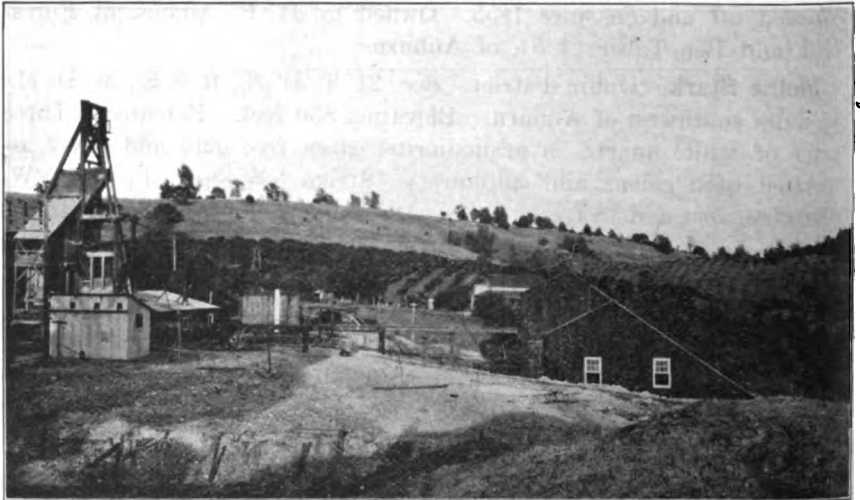
Photo No. 10.—Headframe and mill of the Oro Fino Mining Co., on Bullion No. 1, Ophir District.
