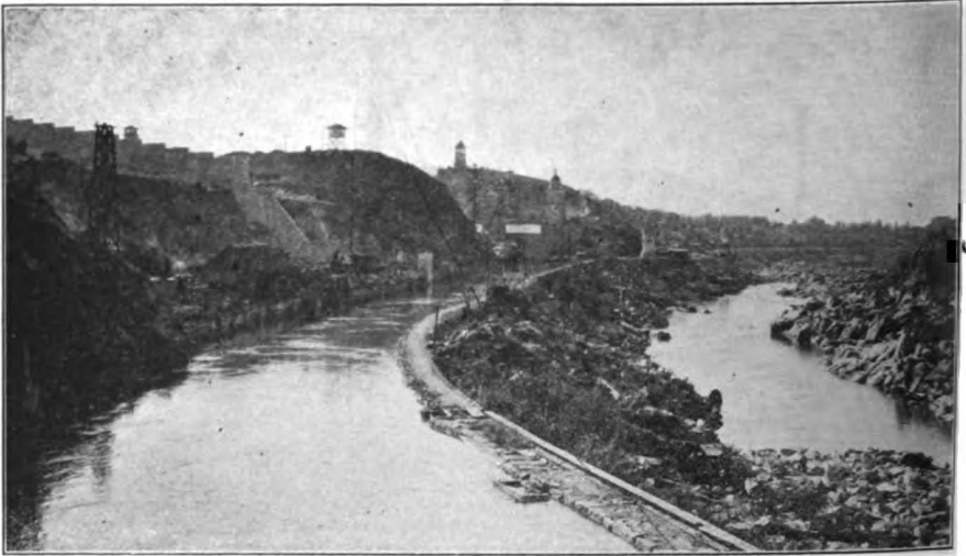
Photo No. 49. View down the American River from the Folsom Prison dam, showing granite outcrops along the river bed and along cuts made for the outlet canal. The prison buildings and walls were built of granite blocks by convict labor.
