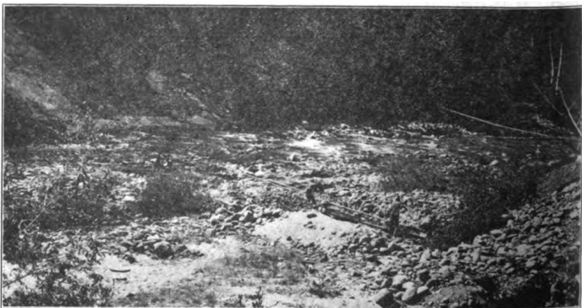
Photo No. 27. Sluicing bench gravels on the south side of the North Fork of the American River, one-half mile below the Iowa Hill bridge, east of Colfax. A small gas engine is used to pump water from the river into the sluice boxes.
