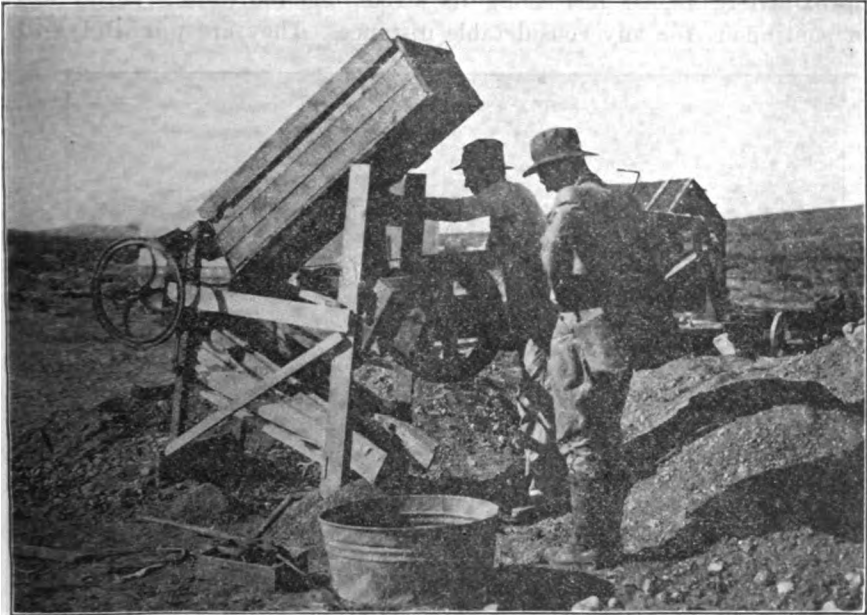
Photo No. 20. Home-made, hand-driven, dry concentrator, working scheelite placer ground at Atolia. Photo by C. A. Waring, March, 1916.
