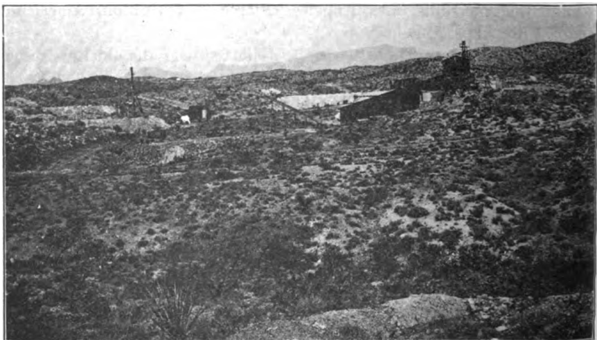
Photo No. 37. New 50-ton mill of the Louisiana-California Mining Co. The head-frame of the 900-ft. shaft is seen at right extending above the top of the mill. The 200 ft. shaft is indicated by the headframe and dump at the left.
