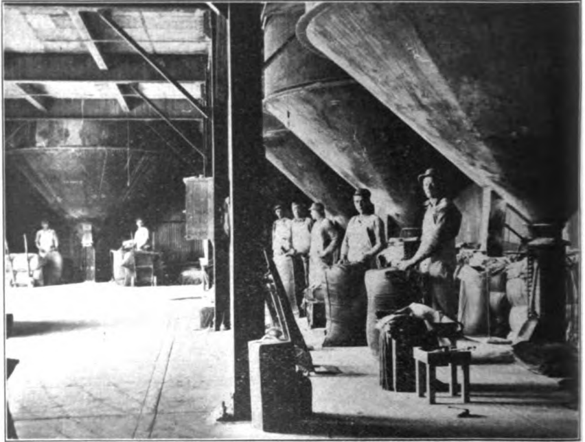
Photo No. 38. Sacking concentrates at the plant of the Pacific Coast Borax Company, Death Valley Junction.
