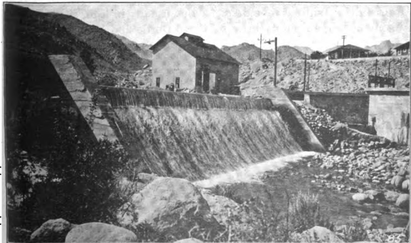
Photo No. 26. General view of Station No. 5 of the Southern Sierras Power Co., on Bishop
