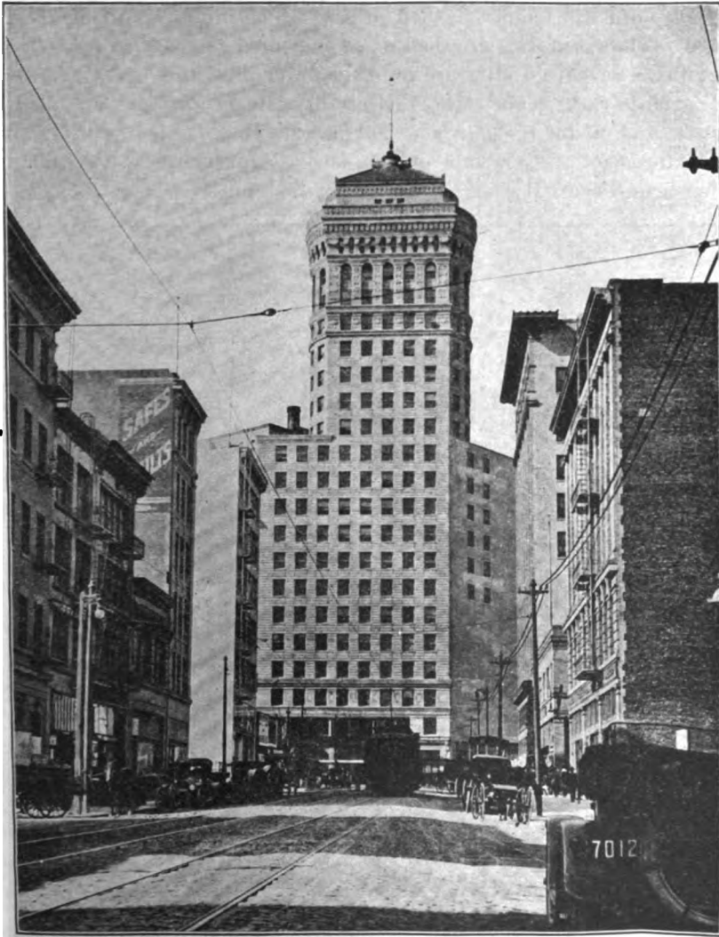
Photo No. 3. Hobart Building, San Francisco, faced with architectural terra cotta, manufactured by Gladding, McBean & Co. plant at Lincoln, Placer County. Photo by Walter W. Bradley.
