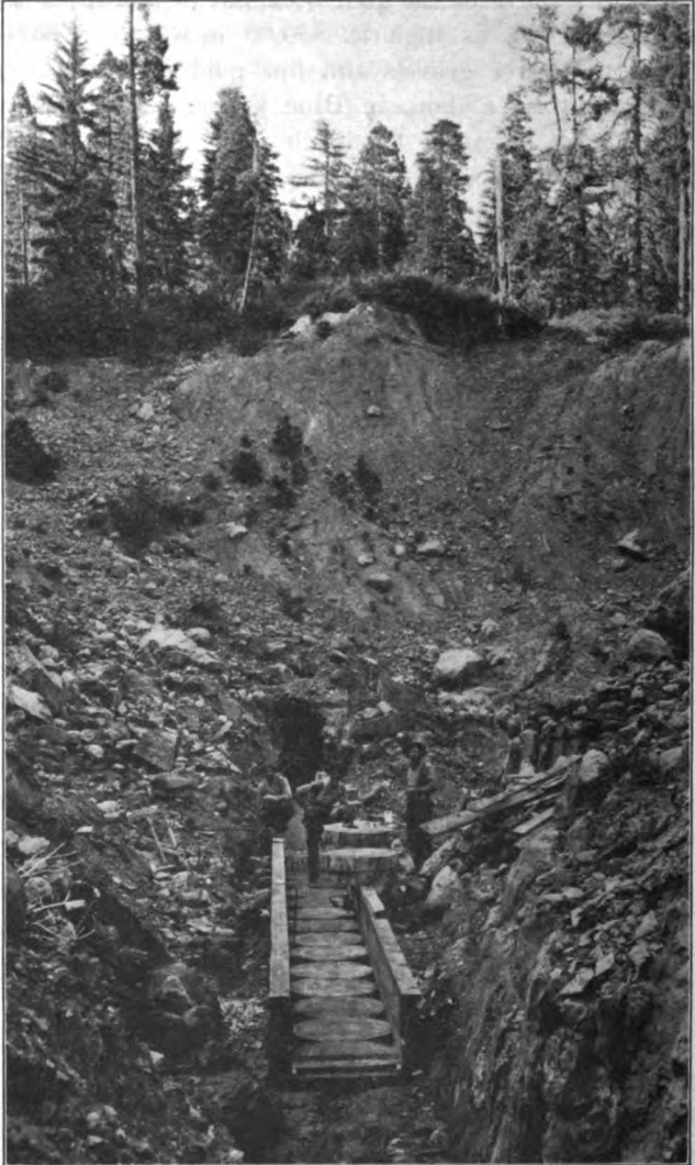
Photo No. 24. Installing sluice boxes for hydraulicking at the Pine Nut Mine, Canada Hill District, Placer County.
