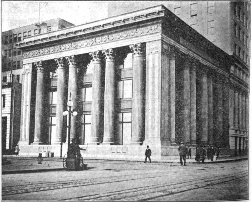
Photo No. 4. Headquarters of Firemen's Fund Insurance Co., San Francisco, faced with architectural terra cotta manufactured by Gladding, McBean & Co. plant at Lincoln, Placer County. Photo by Walter W. Bradley.
