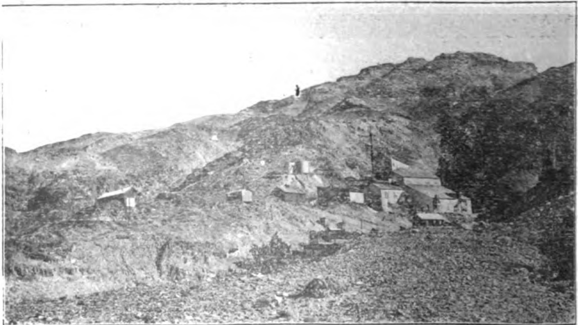
Photo No. 46. Keane Wonder Mill. View northeastward.
