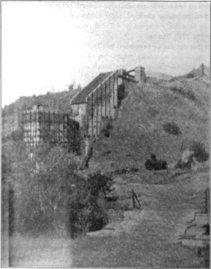
Furnace and condensers, Klau Quicksilver Mine, San Luis Obispo County.
