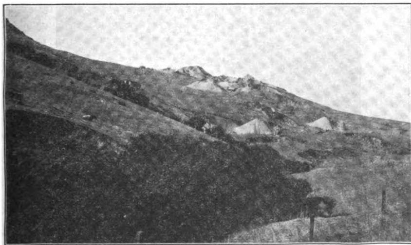
Limestone Quarry of the Union Sugar Co., southwest of Lompoc.
