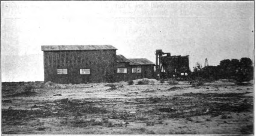
Photo No. 33. Custom Mill at Goffs, built by H. I. Reynolds for concentrating tungsten ores of the Signal and New York Mountains districts.
