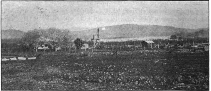
Photo No. 12.—View northeastward from a bridge two miles south of Pentz showing hydraulic tailings from the old Cherokee hydraulic mine.
