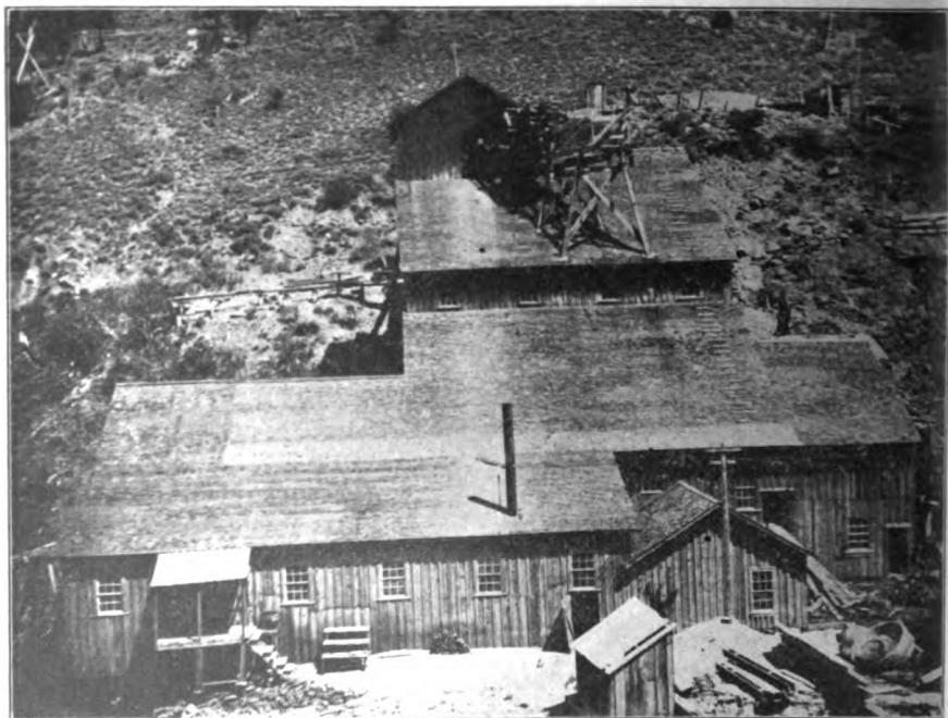
Photo No. 5. Old Alpine Mill, on East Carson River, now used for power house by the Curtz Consolidated Mines Co.
