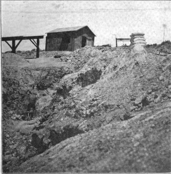
Photo No. 10. Open cut work at original strike at Goldstone Mine. Shaft in background.
