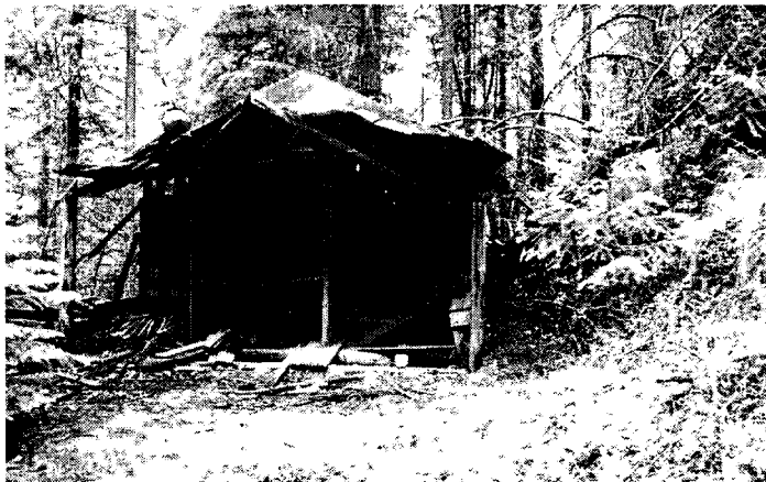
FIGURE 42: SIMPLE WOOD BUILDINGS, MOST AT LEAST PARTIALLY COLLAPSED, DOCUMENT THE SPARTAN LIVING ARRANGEMENTS AT EVEN A MODERATELY SUCCESSFUL MINING OPERATION (RRNF SITE 702-D).
