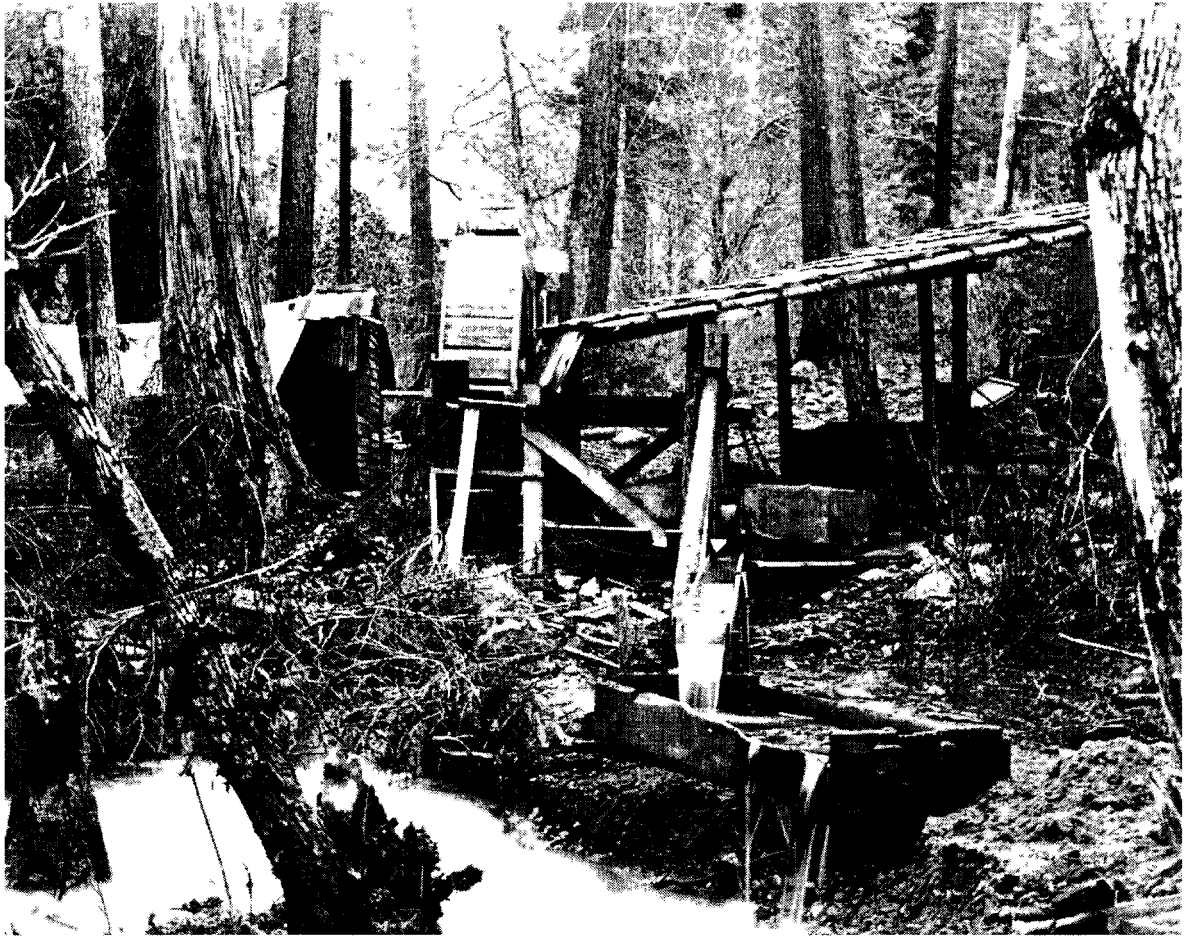
FIGURE 20: AN EARLY WATER-POWERED ARRASTRA, SERVED BY A SIMPLE WOODEN FLUME (TO THE RIGHT), GROUND ORE, WHICH WAS THEN SLICED THROUGH THE RECTANGULAR BOX IN THE FOREGROUND (JOSEPHINE COUNTY HISTORICAL SOCIETY COLLECTION).
