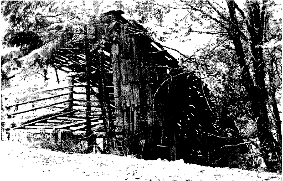
FIGURE 38: VIEW FROM UPPER ELEVATION OF THE STEAMBOAT STAMP MILL (RRNF SITE 603).
