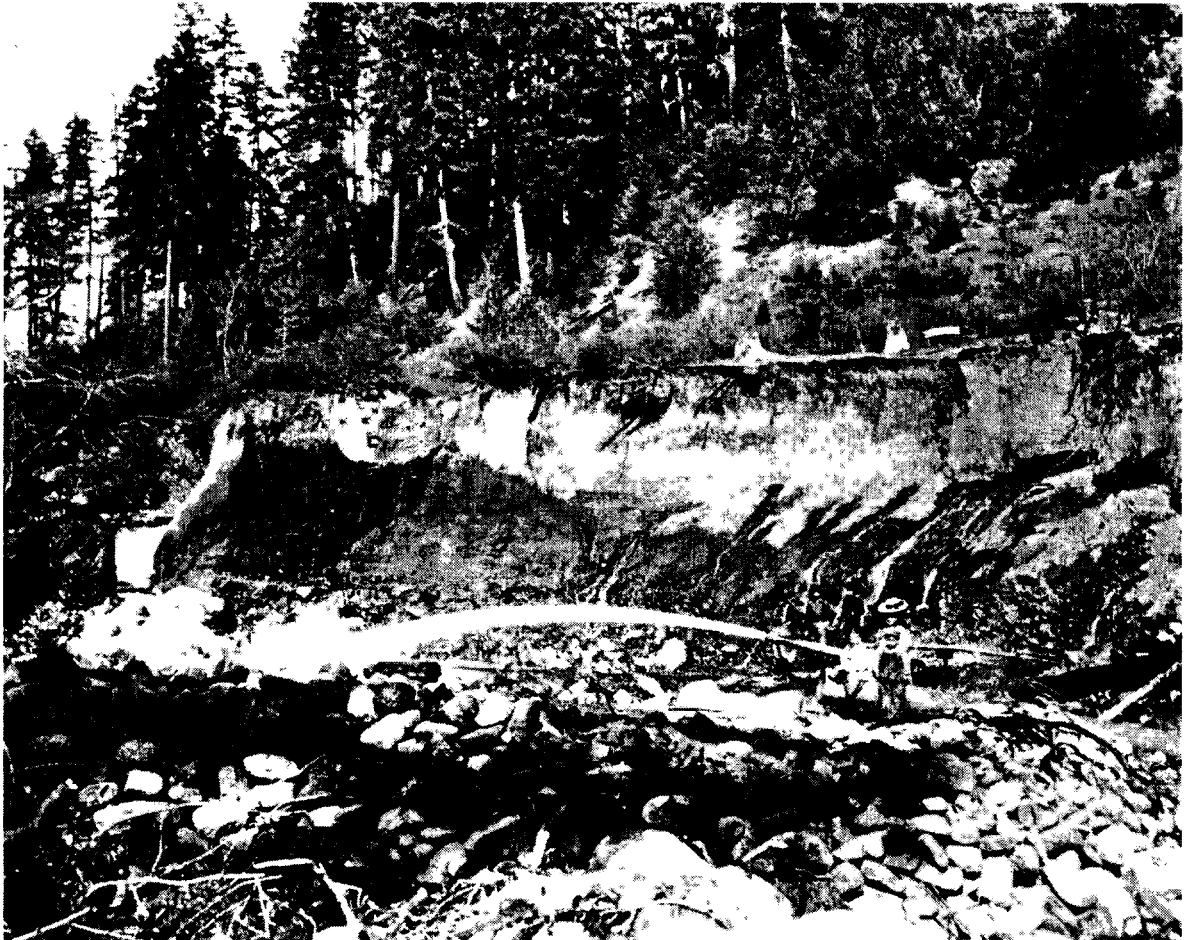
FIGURE 13: LARGE-SCALE HYDRAULIC MINING DRAMATICALLY CHANGED THE LANDSCAPE, CUTTING AWAY THE BANKS OF STREAMS AND SENDING SILT, ROCK AND OTHER DEBRIS DOWNSTREAM. STILL, THE EXCITEMENT OF THE GIANT PROVIDED PRIDE AND ATTRACTION FOR THE FAMILIES OF THE MINERS, BRINGING THIS WELL-DRESSED MOTHER AND HER TWO CHILDREN OUT FOR A VISIT, c1900 (PERCY BOOTH PHOTO, JOSEPHINE COUNTY HISTORICAL SOCIETY COLLECTION).
