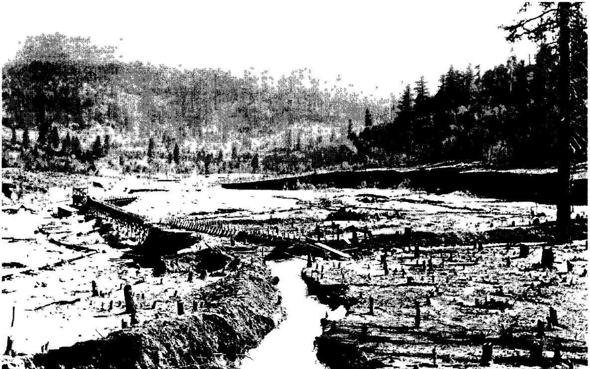
FIGURE 16: FLUME OF THE SEATTLE MINE COMPANY, ON ELLIOTT CREEK. EXTENSIVE FLUME AND DITCH SYSTEMS, SUCH AS AT THIS JOSEPHINE COUNTY MINING OPERATION, WERE REQUIRED TO CHANNEL AND RE-DIRECT THE AREAS OFTEN LIMITED WATER SUPPLIES (PERCY BOOTH PHOTO, JOSEPHINE COUNTY HISTORICAL SOCIETY COLLECTION).
