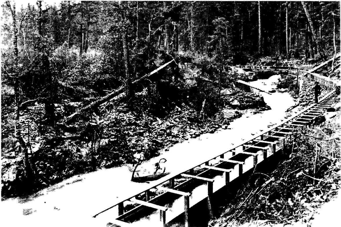
FIGURE 33: ALTHOUGH EXTENSIVE WOOD FLUMES WERE BUILT IN THE AREA, OFTEN ON TRESTLES SUCH AS IN THIS VIEW OF A 19 TH CENTURY JOSEPHINE COUNTY MINE, MOST WERE EITHER SCAVENGED FOR LUMBER OR FUEL OR HAVE SIMPLY COLLAPSED AND DECOMPOSED (BOOTH PHOTO, JOSEPHINE COUNTY HISTORICAL SOCIETY COLLECTION).
