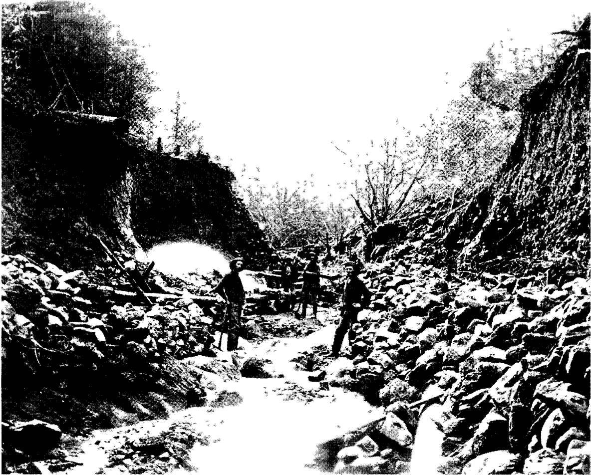
FIGURE 12: SUMMER “HYDRAULICKING” AT THE LAYTON MINE, FERRIS GULCH, APPLGATE VICINITY, c1890 (JOSEPHINE COUNTY HISTORICAL SOCIETY COLLECTION).
