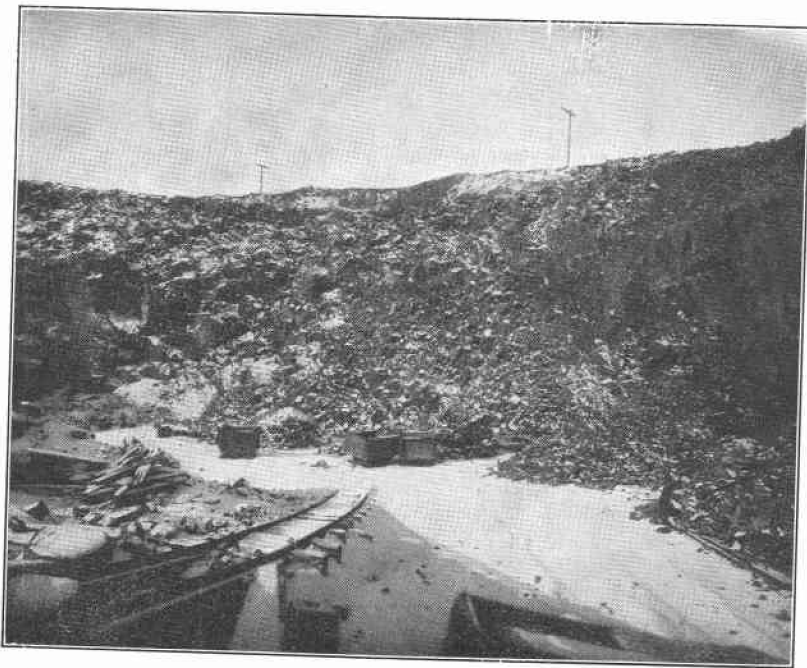
BASALT QUARRY, BAKER, OREGON—USED IN CONNECTION WITH CONSTRUCTION OF BITULITHIC PAVEMENT.
